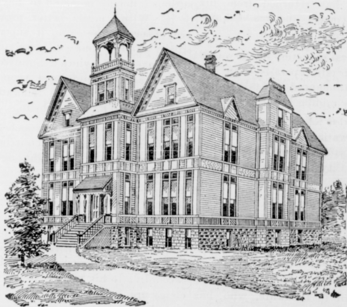
Building in Course of Construction.
