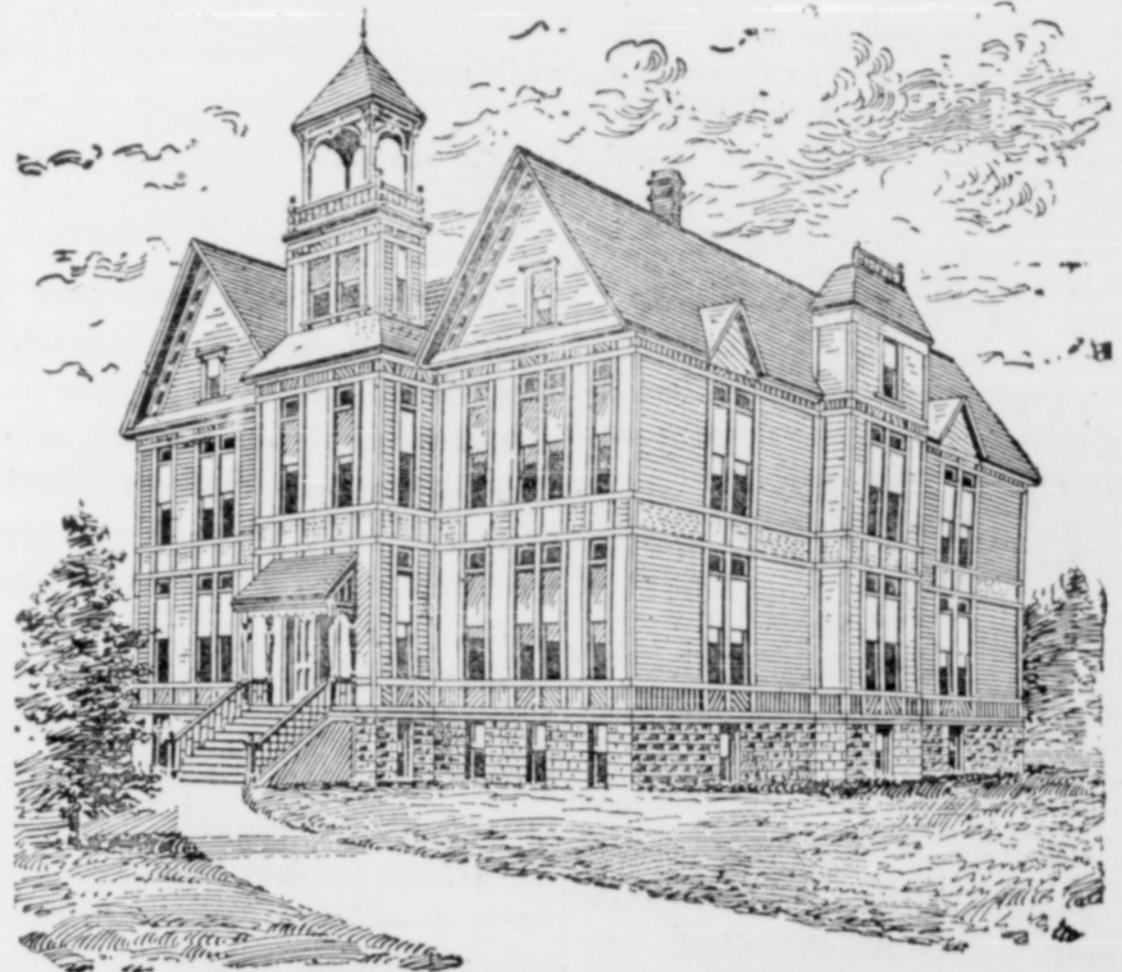
Building in Course of Construction.
