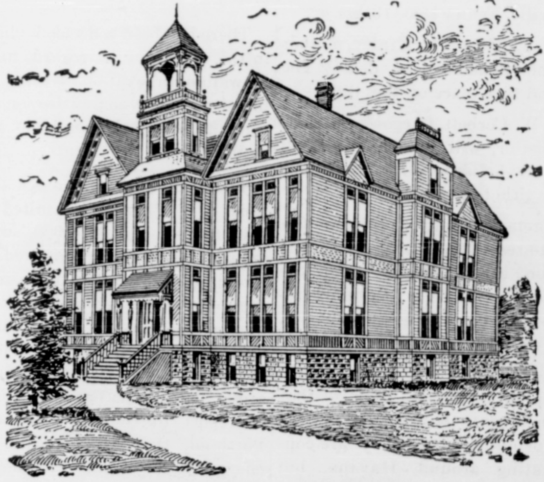
Building in Course of Construction.
