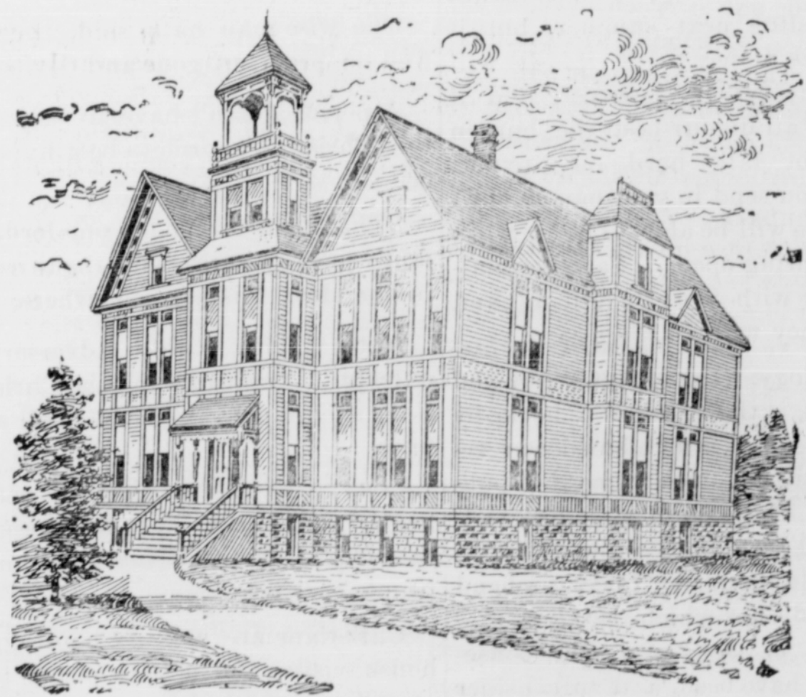
Building in Course of Construction.
