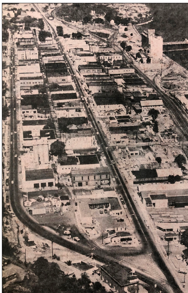
Downtown The Dalles main streets, paralleling the Columbia River and the Union Pacific Railroad tracks, are shown in this aerial photograph by Mell Olmstead, looking west — or downstream. Second Street, the westbound arterial, is on the right, flanked by rail and river, with the Port of The Dalles dock and grain elevator. On left is Third, eastbound arterial, with main business blocks between. — The Dalles Daily Chronicle , June 30, 1961
