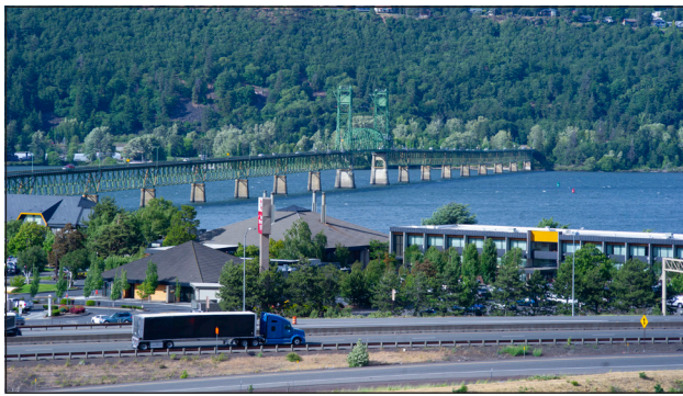
Progress is being made to establish an Oregon-Washington ownership of a new bridge over the Columbia River in Hood River, replacing the existing bridge, above, which is 100 years old.
