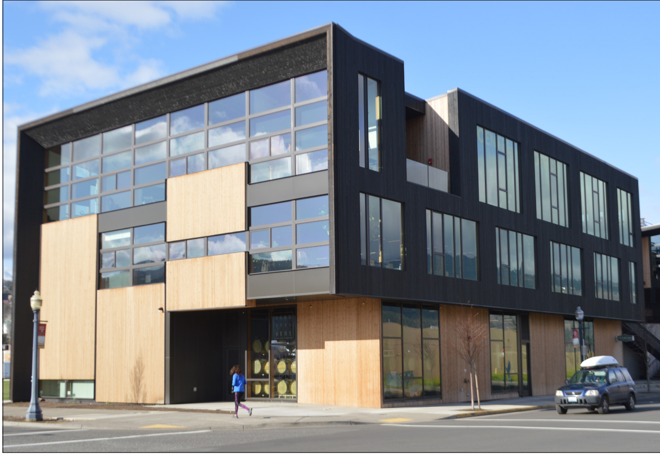
Outpost, at Second and Portway avenues in Hood River, earned a national design award from WoodWorks.
