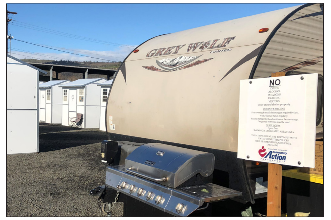
A staff volunteer occupies the trailer at right when the pallet homes in The Dalles are in use. A list of rules are posted for those using the site. Mark B. Gibson photo
