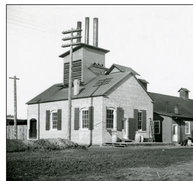
Early electric power would light a few bulbs for a few hours each evening in the homes of The Dalles. Power came from this wood-fired steam plant at the corner of First and Laughlin Streets. Photo courtesy
