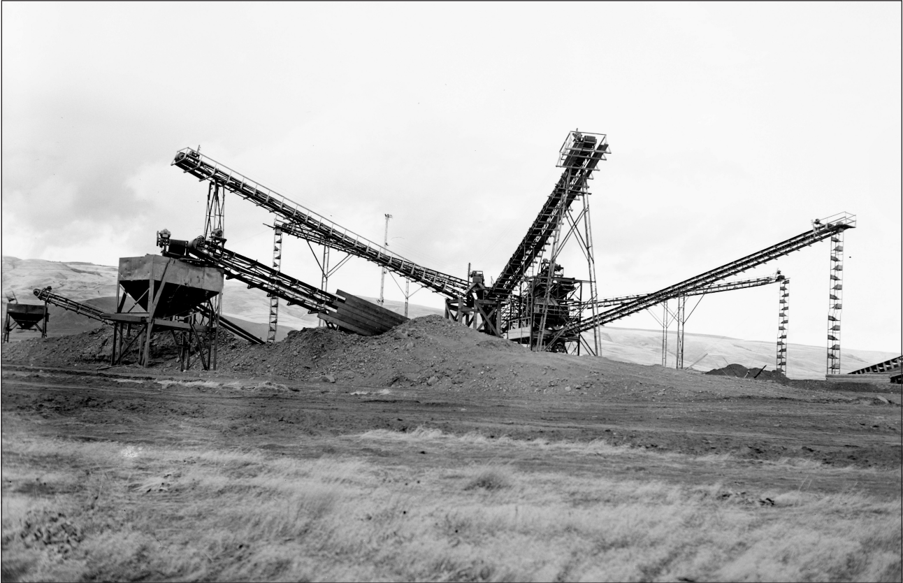
A sprawling sand and gravel plant sorts and prepares gravel and sand for use in the construction of The Dalles Dam on Nov. 1, 1953. Scanned from a 5-by 5-inch black and white negative.
