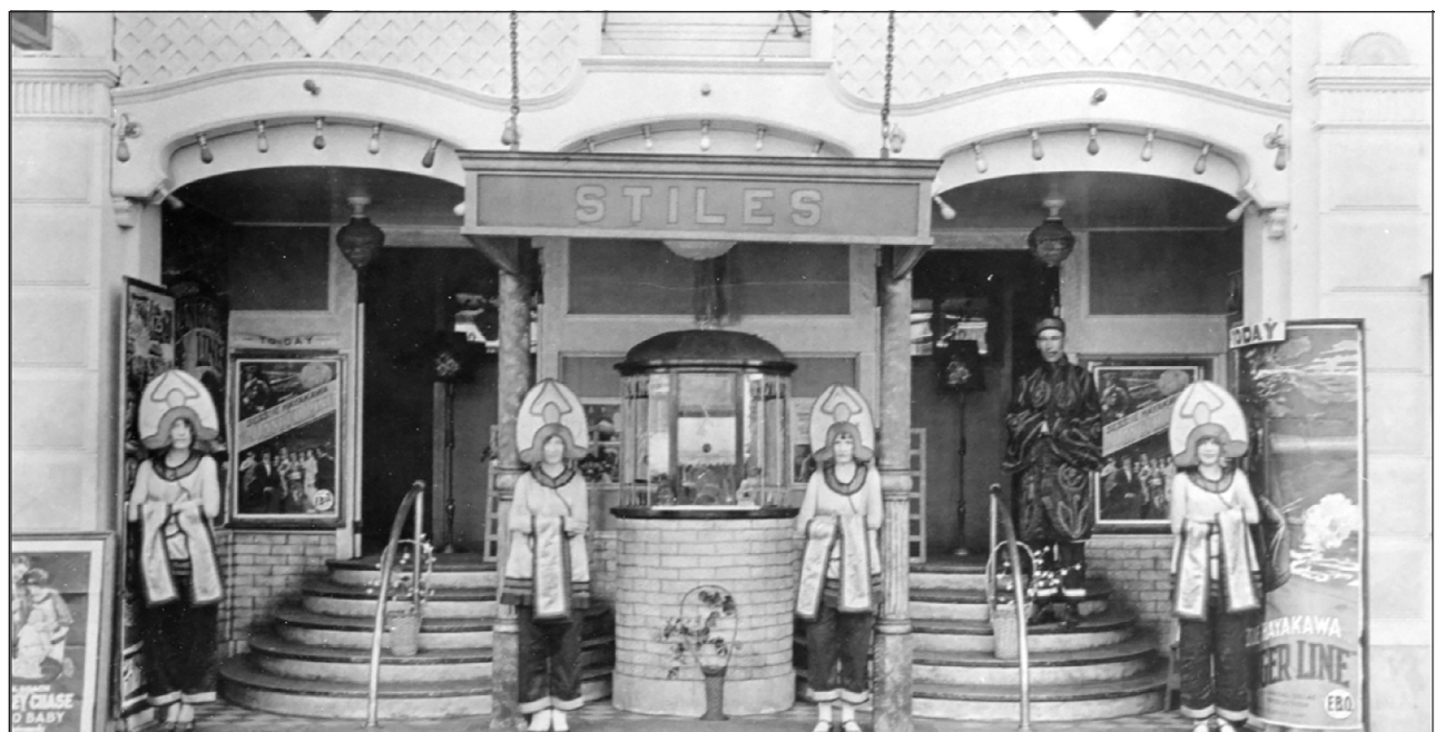
The Stiles Movie Theater, located on the 200 block of 2nd Street in 1925.
