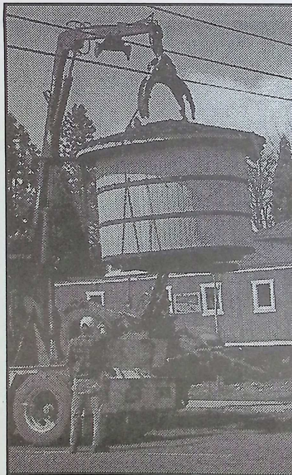
HEY ... Watch out for those wires !!!! A water tower was recently added to the Caboose Museum, to keep things cool.
