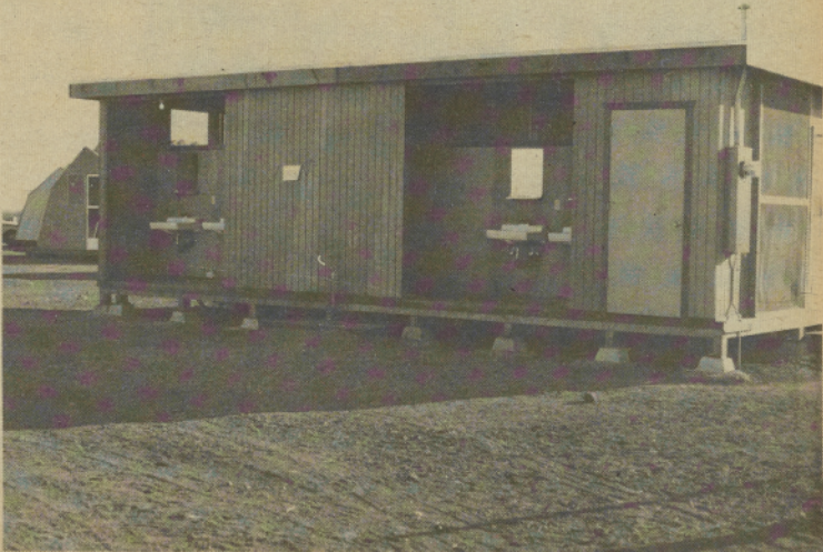
Madison Camp has four bath and toilet units. Each unit has eight showers and eight toilets. These facilities are cleaned twice a day.
