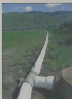
Gated pipe installed; replacing flood irrigation in both Baker Valley and Burnt River.
