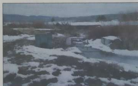
One sill/wing diversion structures on Camp Creek; Juniper bank stabilization.
