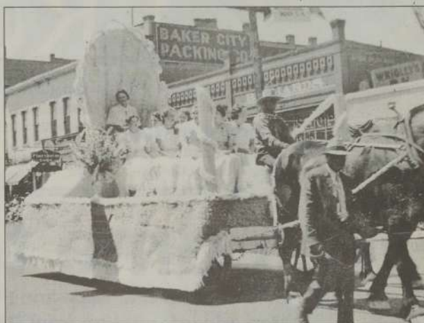
Photo from Baker County Library, Baker City
