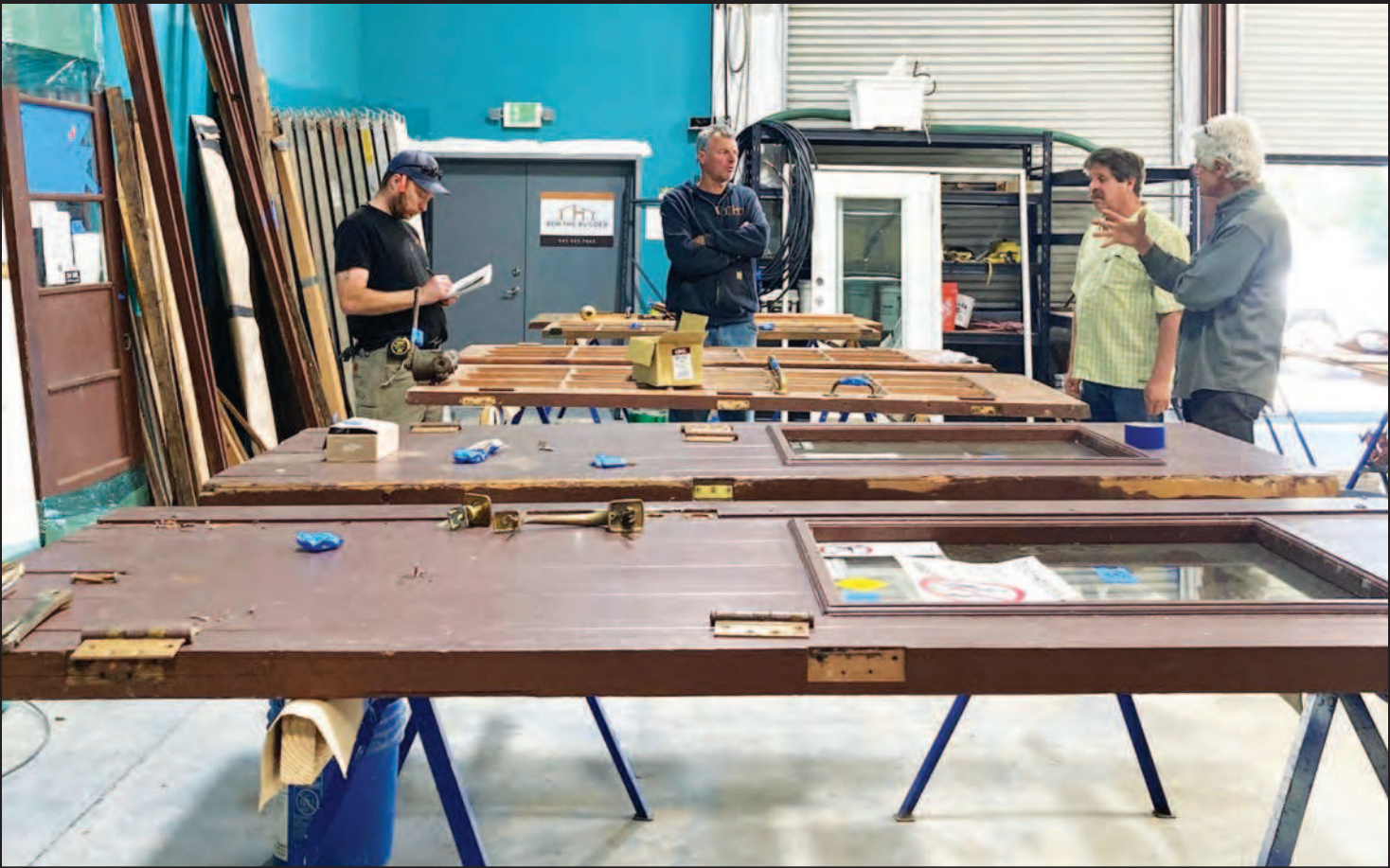
Restoring the doors of the Chateau above is Ryan, Ben the Builder contractor (left); Mark Friis, Ben the Builder contractor; George Kramer, historic preservation consultant; and Jay Treiger, door restoration specialist from Ben the Builder. The photo on the right is one of the Chateau balconies that was removed in 1950.
