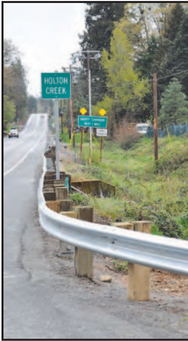
Hwy. 199 at Holton Creek where the bridge will be built starting Tuesday, April 12.
