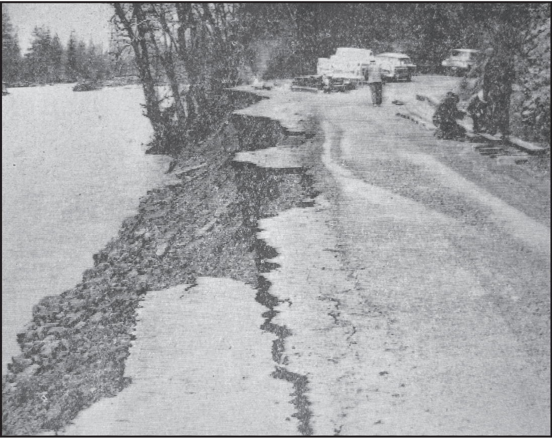
At Takilma Road and Hogue Hill the park crew builds up a ditch to widen the remaining lane of a two lane road.
