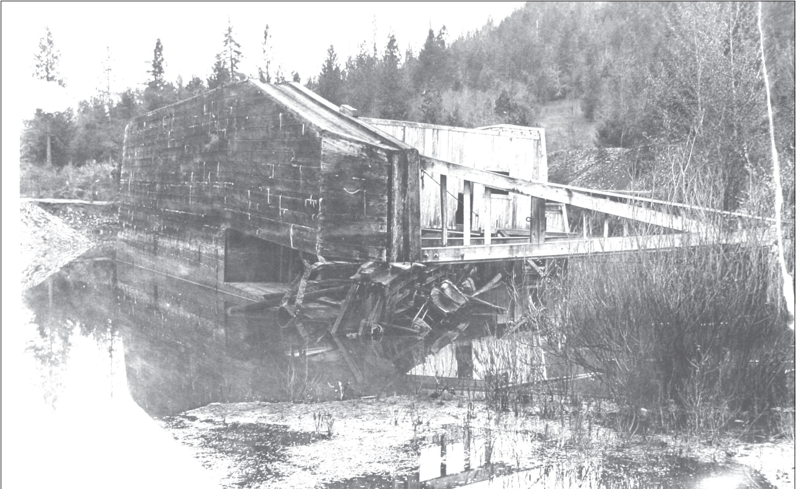
The bottom of the dredge faces to the left and a lift arm for the bucket-ladder faces to the right. Some of the buckets can be seen lying in the water. The other half of the boat is under water. Kerbyville Museum collection.
