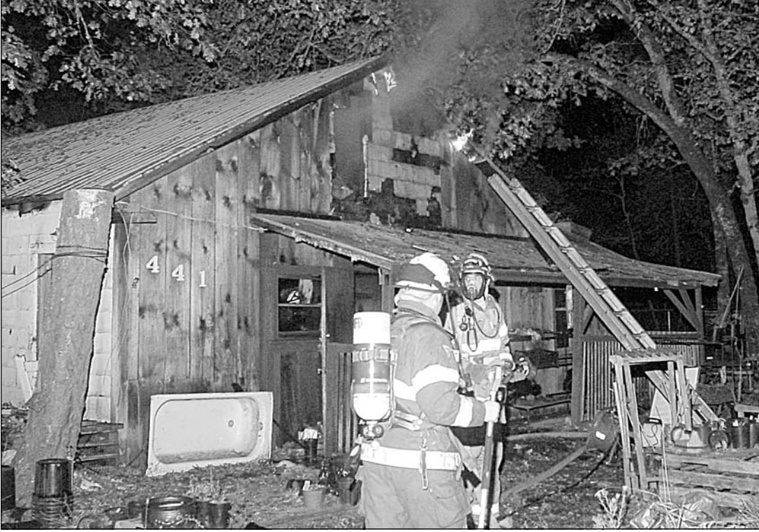
Illinois Valley Fire District (IVFD) personnel responded with two engines and a tender on Friday, Oct. 23 to a 7 p.m. alarm at the former Family Tree Nursery on S. Junction Avenue. Crews fought the fire for some two hours. Rural Metro and Grants
