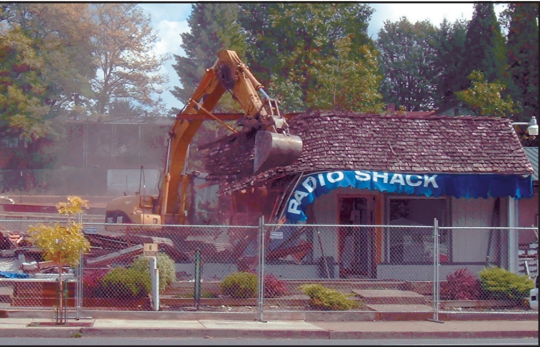
Making way for a new CJ Video Mart/Radio Shack in Cave Junction meant that the former building was demolished last week. The new structure, with 4,000 square feet of space, is double the size of the old one. Although videos temporarily aren't being rented, items are being sold in the new structure. It's hoped that concrete work will be finished next week. The main contractor is A Better Builder; Doug Kendall is the architect. (Dusty Rhodes photo)
