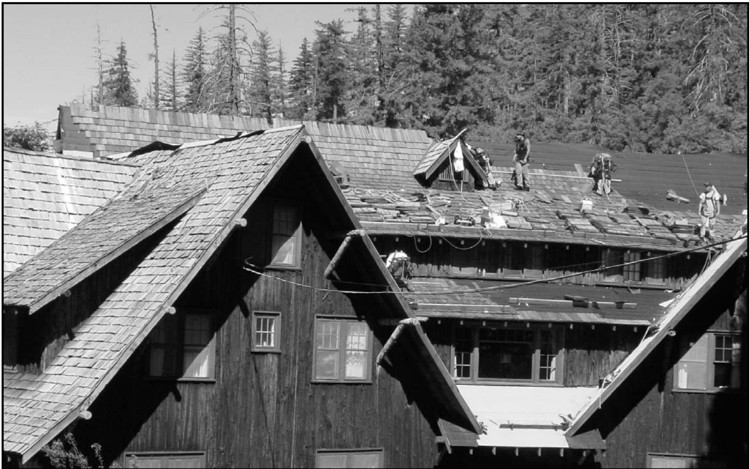
WHAT'S SHAKIN' AT CHATEAU? New cedar shake shingle and fire-retardant material beneath, that's what. Harnessed and roped, workers maneuvered atop the steeply pitched roof of the historic Chateau at Oregon Caves National Monument. The picturesque lodge
