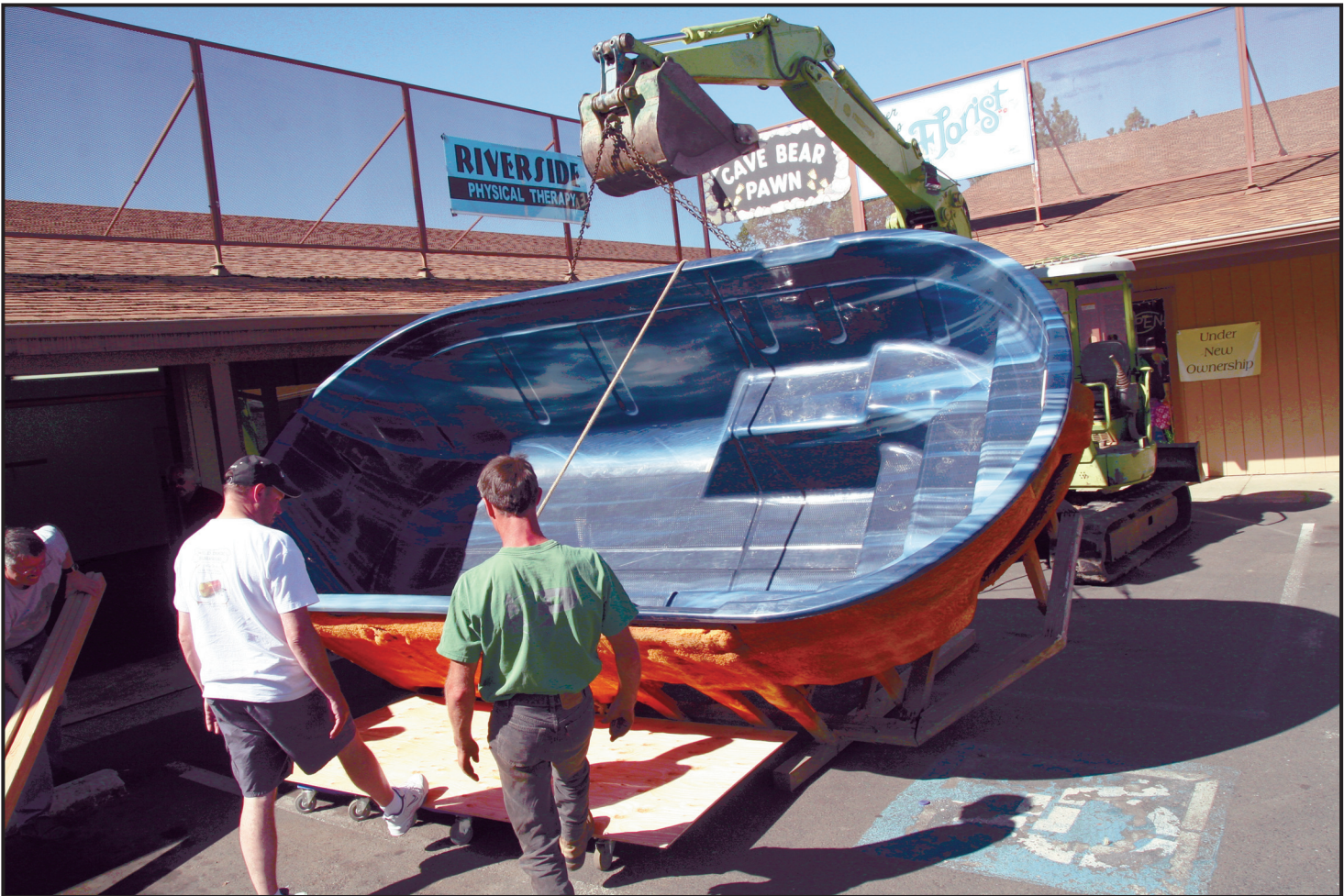
RIVERSIDE PHYSICAL THERAPY in Western Plaza in Cave Junction took delivery of a large tub for use in low-impact exercise and physical therapy. Installation of the pool, which is 8-feet wide and 16-feet long, required that a double door and window be temporarily
