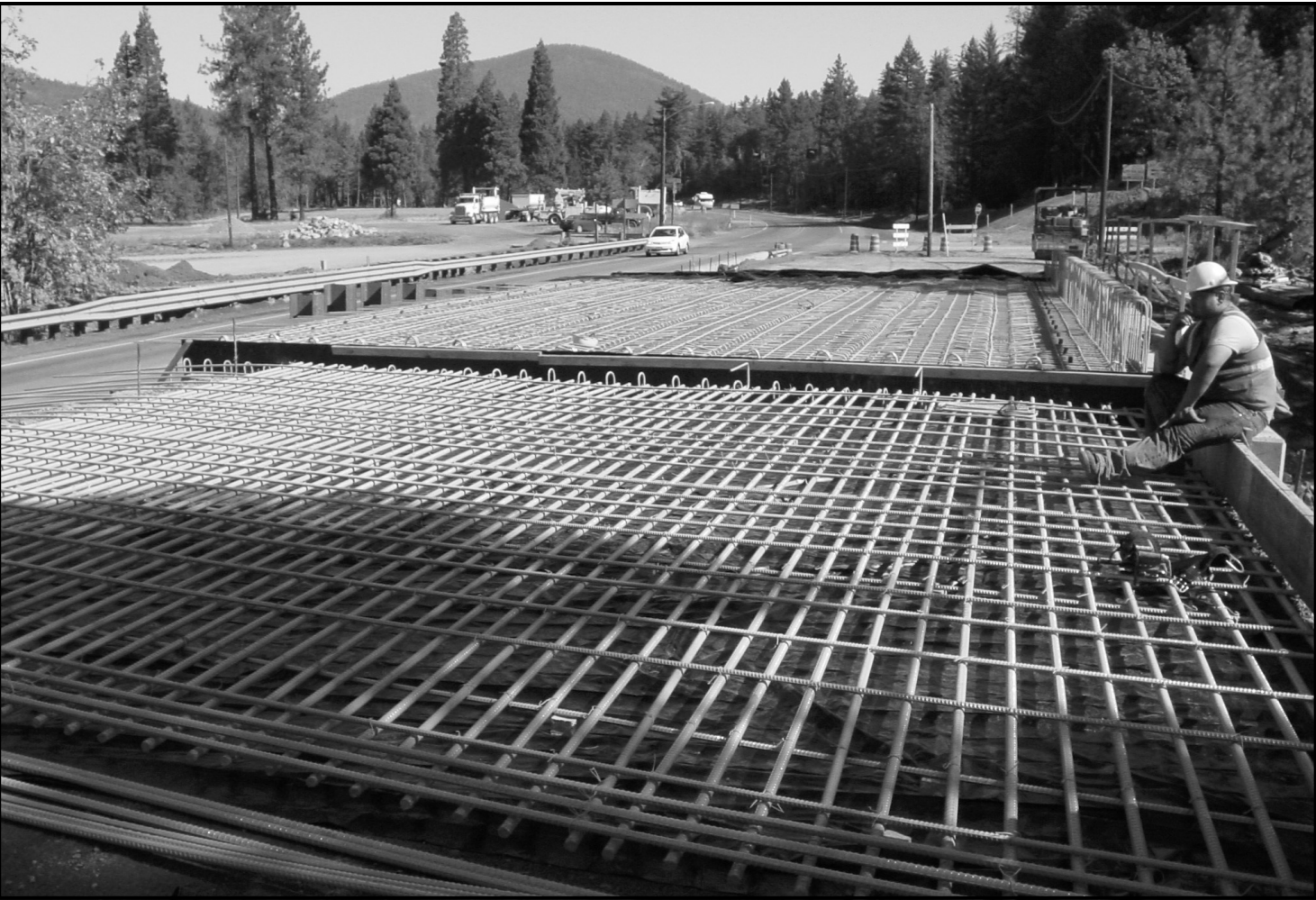
STEEL YOURSELVES -- At Hwy. 199 and Laurel Road on the north edge of Cave Junction, work to replace the bridge over George Creek is progressing. The project is valued at $5.5 million, said Oregon Dept. of Transportation. In connection with the bridge replacement, the highway is being widened from approxi-
