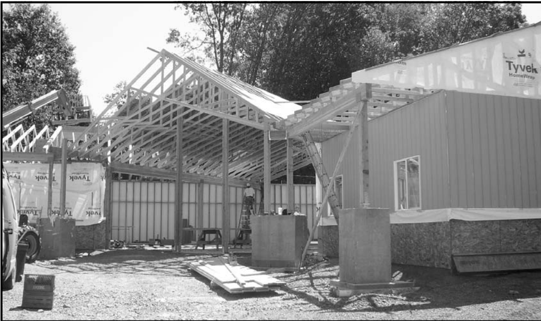
CONSTRUCTION CONTINUES in Cave Junction on new quarters for CJ Video Mart/Radio Shack , owned and operated by Bill & Chris Coultas. The work is being done by A Better Builder , of Cave Junction. The new facility will more than double the size of the store. (Photo by Illinois Valley News )
