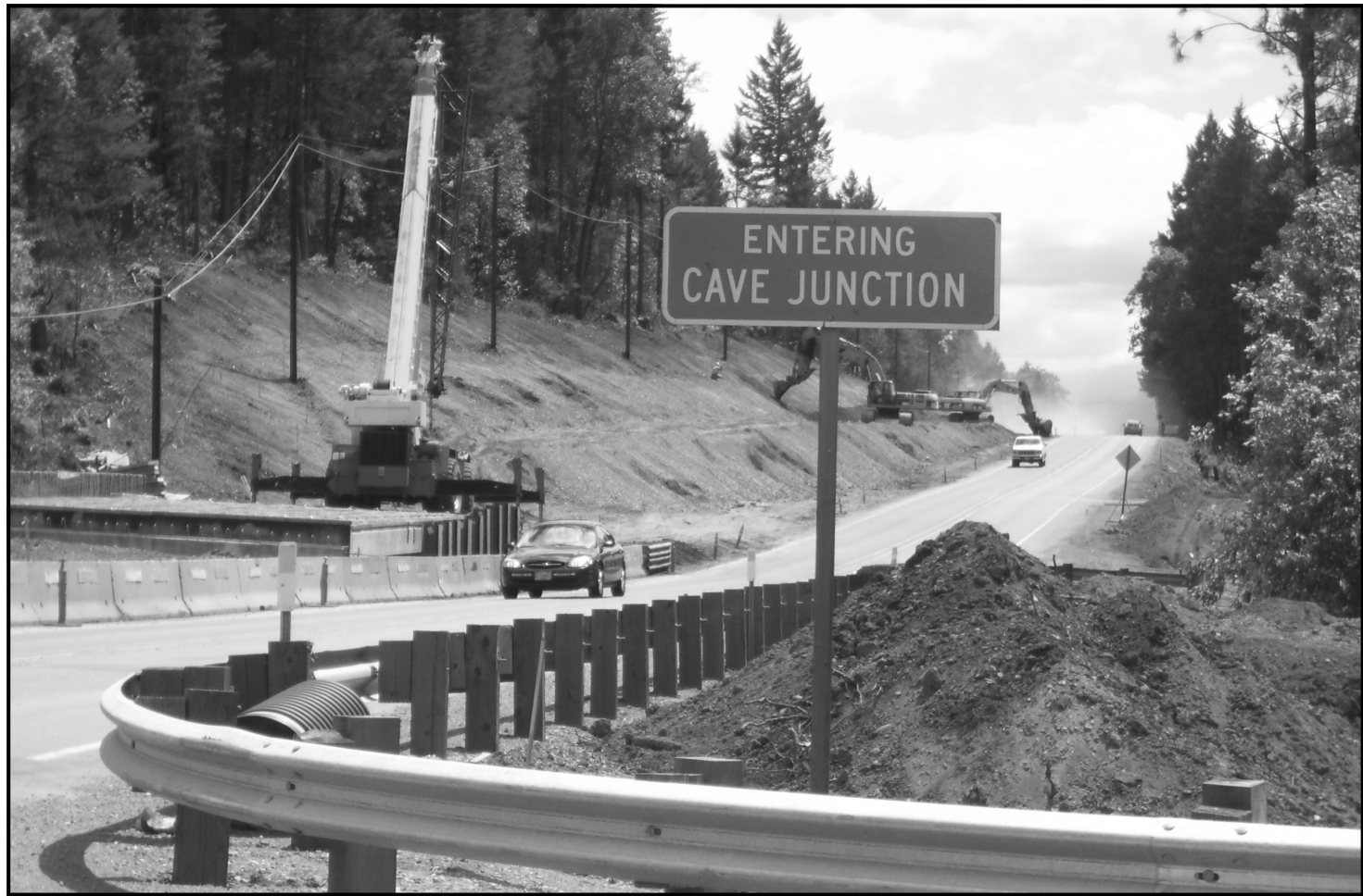
WIDENING OF HWY. 199 continues at the north end of the city of Cave Junction. The $12.5 million project is being done by Copeland Paving of Grants Pass. The work involves widening the road from a point just north of Laurel Road south to Wild River Brewing & Pizza Co. (Photo by I.V. News)
