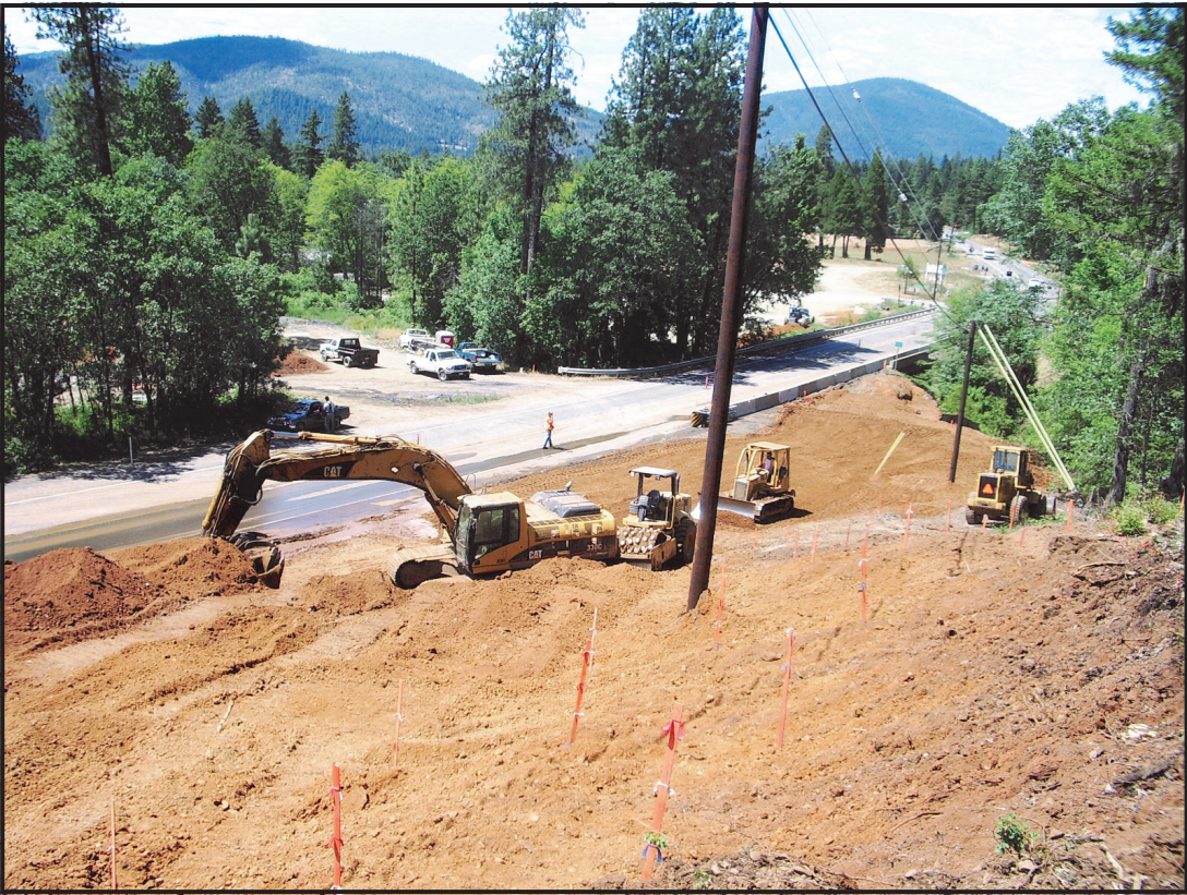
Copeland Paving & Asphalt has the $4.5 million contract with ODOT to widen Hwy. 199 from the Laurel Road area, north to Wild River Brewing & Pizza Co. (Photo by I.V. News)
