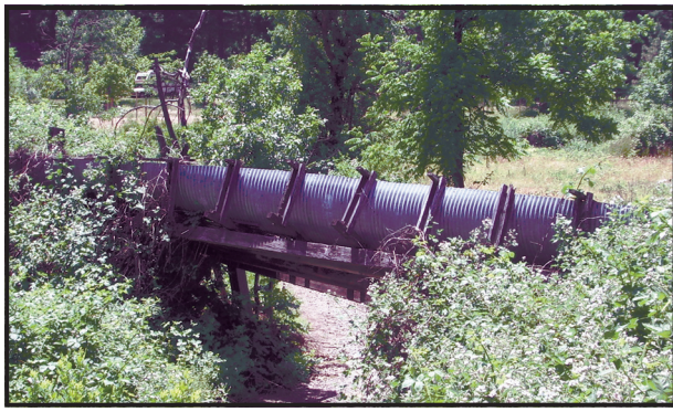
A remnant of the Kerby Ditch system
