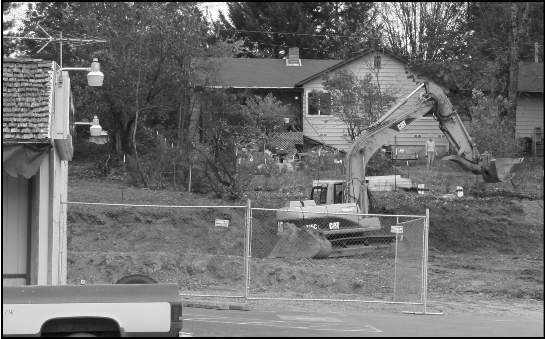
A NEW RADIO SHACK and CJ Video Mart is scheduled for completion possibly by July. Excavation is under way for the new building which will be twice the size of the current structure, said Chris Coultas, co-owner with her husband, Bill. The existing building will be razed. The project will result in the corner of Redwood Hwy. and E. River Street being open for customer parking. (Photo by 'Illinois Valley News)
