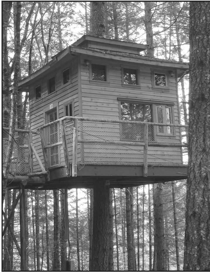
This view shows the 'Shitake,' one of two accommodations. Note tree going through the middle. (Photo by Scott Jorgensen/Illinois Valley News')
