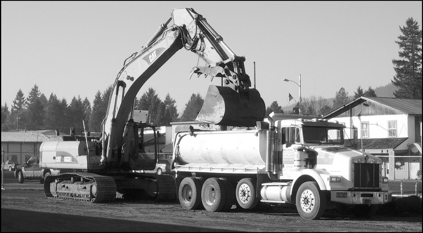
HOME VALLEY BANK will relocate this year to the site in Downtown Cave Junction of the former Select Market. Site preparation by Copeland Sand & Gravel con-
