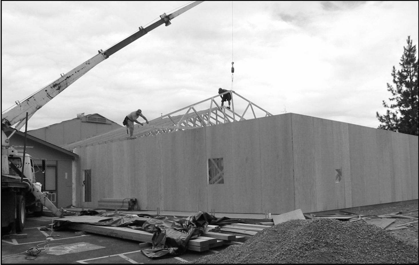
AN EXPANSION PROJECT AT Illinois Valley Senior Center on E. River Street in Cave Junction continues to progress. The addition of a 40-by-60-foot room is needed to accommodate growing programs and activities, which have outgrown the available space. General
