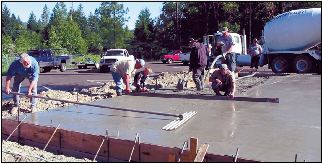
ILLINOIS VALLEY SENIOR CENTER is being expanded with addition of a 40-by-60-foot room because of the need for more space to accommodate programs and activities. Meidinger Concrete Construction poured the slab last week. The general contractor for the $300,000 project is JDB&S Raymond Inc. It and Meidinger are donating some of the work. Approximately $110,000 has been raised through monthly breakfasts, thrift shop sales and bingo proceeds, and there is a need for donations from $1 up to handle finishing, after framing and roofing, including windows, doors, fire sprinklers and electrical needs. Some valleyites have invested $1,000 each in the project. For more information phone 592-6888. (Photo courtesy of Jess Goldtrap)
