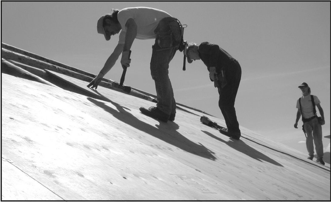
RAISING THE ROOF was the order of the day recently as volunteers placed plywood sheets atop the pole structure that will be used for a farmers market opening Monday, May 15 at Selma Community & Education Center. The metal roof is to be installed Friday and Saturday, May 19 & 20. Solar panels subsequently will be added and be in operation by mid-June to provide power. (Photo provided courtesy of Selma Community & Education Center)
