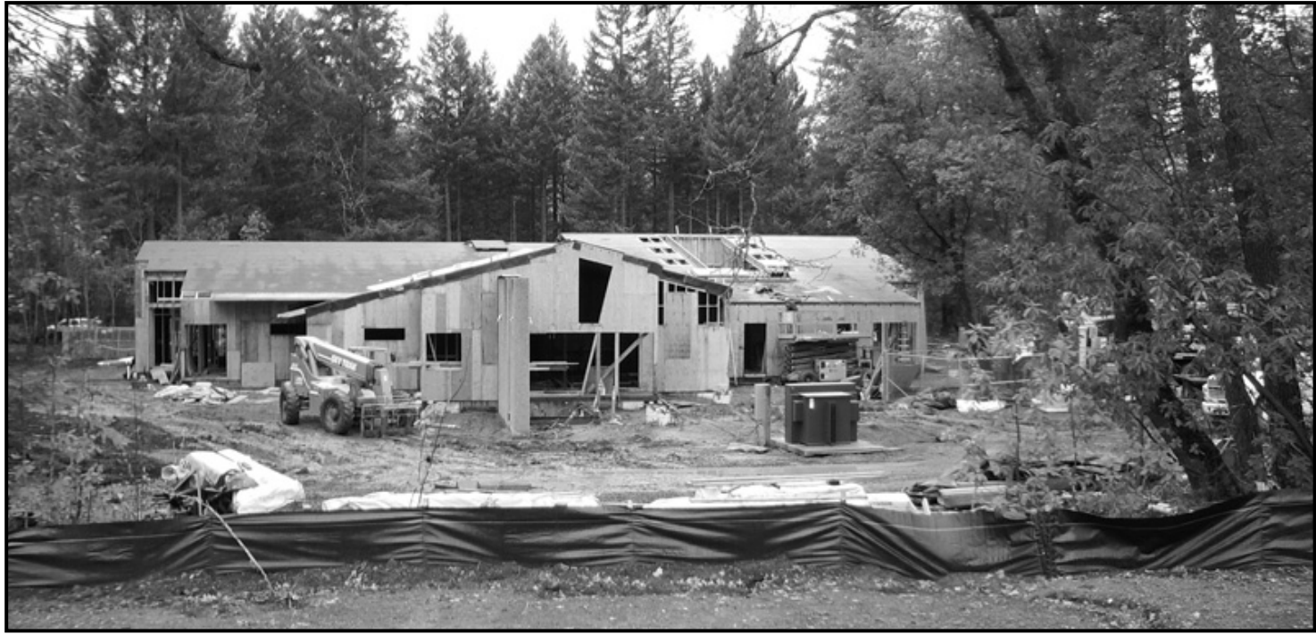
CONSTRUCTION PROGRESS CONTINUES at the north end of the city of Cave Junction on the new Siskiyou Community Health Center (SCHC). This view is from the east side. The clinic, with 10,000 square feet of space, will allow SCHC not only to serve more people, but through a partnership with Three Rivers Commu-
