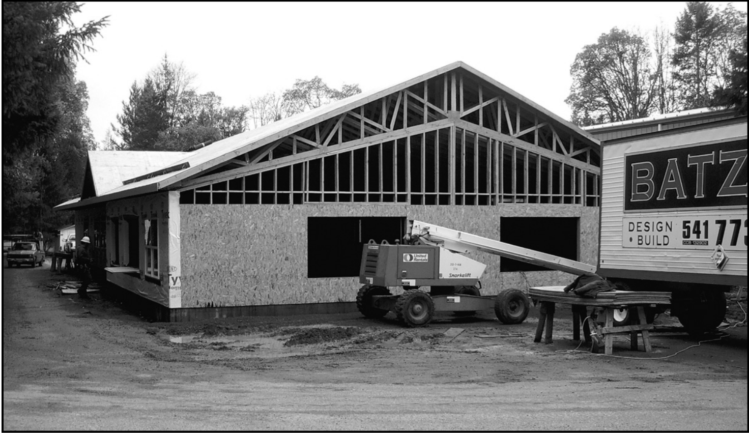
ILLINOIS VALLEY FIRE DISTRICT plans to move into a new administrative headquarters building next to the new Cave Junction Station 1 during the last week of January 2006, said Chief Harry Rich. Batzer Construction, of Medford, is the primary contractor for the single-story building with approximately 5,900 square feet
