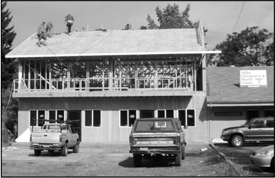
NEW IN CAVE JUNCTION - Work is progressing on a two-story commercial building on Lister Street across from the CJ Post Office. Owner Sally Palmer said, ‘Bruce Donaldson has an excellent crew and they are doing a great job building ahead of schedule. I’m very proud of the building.’ The structure has a total of 3,000 square feet of space. It’s designed to have two businesses downstairs and two residences upstairs. However, a single business is interested in the entire building, Palmer said. (Photo by ‘Illinois Valley News’)
