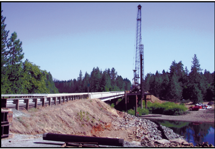
HIGHWAY BRIDGEWORK continues on the three bridges over Illinois River in Cave Junction. The work above is at 'second bridge' near the south end of Westside Road. The $15 million project under Oregon Dept. of Transportation is funded under the Oregon Transportation Investment Act. (Photo by 'I.V. News')
