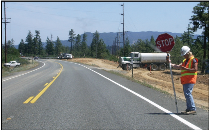
Flaggers are hard at work, as construction on three new bridges is under way in Illinois Valley on Hwy. 199
