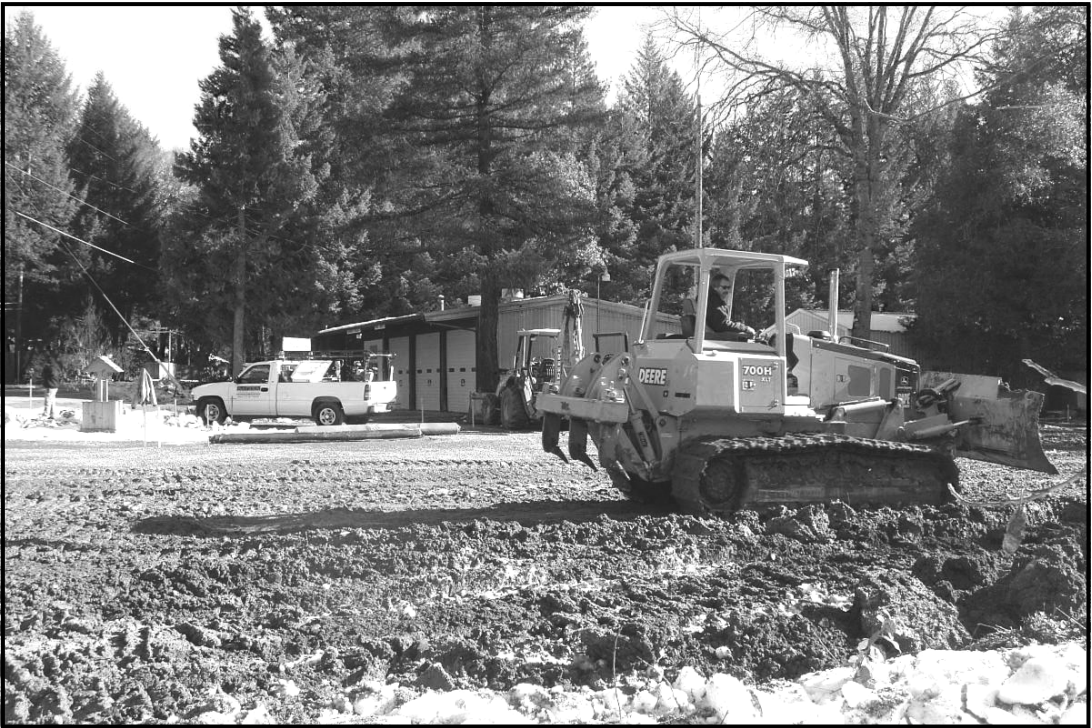
‘DOZER DOING DUTY - Batzer Inc., of Medford, last week began grading a site for a new Cave Junction fire station. The existing building, which is somewhat unsafe, is in the background. Batzer also is working on building new stations in O’Brien and Selma. Funds are from a voter-approved bond issue. (Related story on page 5.)
