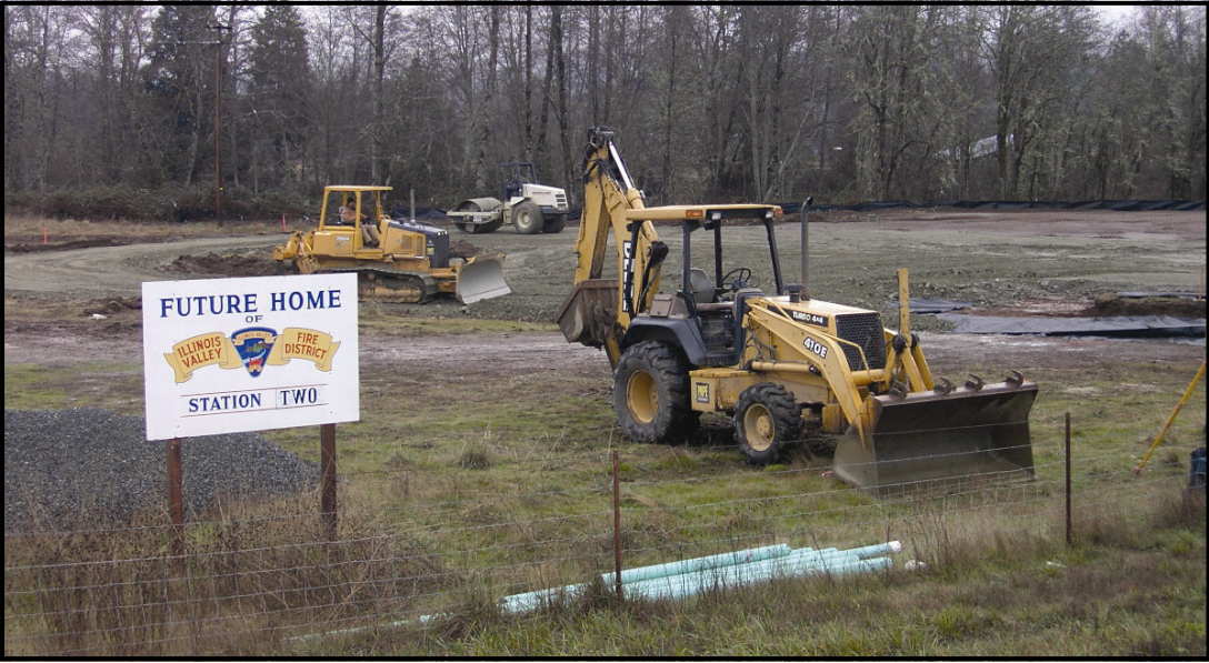
MOVIN’ DIRT FOR NEW STATION - Batzer Construction of Medford has begun preparation work for a new Selma Fire Station on a 3.5-acre site a short distance south of the current station. The new two-story structure will contain approximately 6,300 square feet of space including apparatus bays. The project was to be completed by April 2005, but due to delays caused by a Josephine County ruling that a lift is required under ADA, the completion date is uncertain. The new station is funded through a bond issue approved by district voters.
