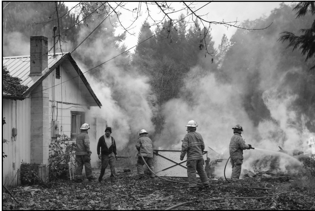
ESCAPED DEBRIS BURN - Contractors burning the remains of a barn that they had knocked down in the 300 block of S. Old Stage Road found that the fire was willing to also burn an adjacent house. The alarm was sounded Thursday, Nov. 18 at approximately 11:04 a.m., and Illinois Valley Fire District firefighters responded to quickly extinguish the flames.
