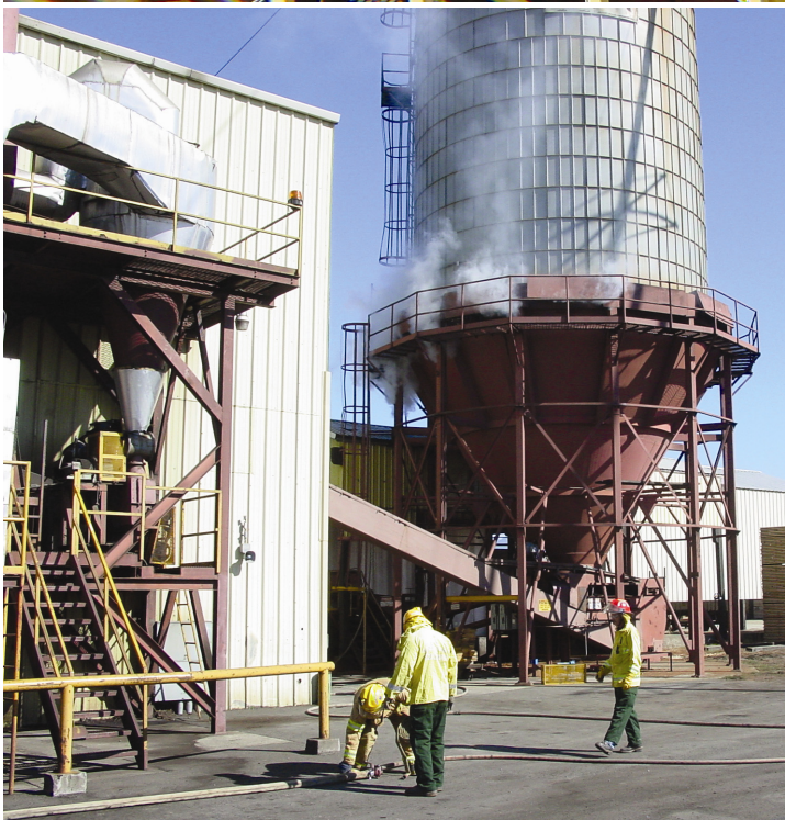
SMOULDERING SILO - Illinois Valley Fire District (IVFD) firefighters responded to a silo fire at Rough & Ready Lumber Co. on Saturday, Oct. 16. The silo contains fuel for a boiler. Despite a volume of smoke, there was not much fire and firefighters contained it. No damage was reported. Firefighters had to haul hoses up 30 feet to combat the blaze. Another alarm for the same problem occurred late Monday afternoon, Oct. 18, but it was quickly handled. (Photos by Dale and Elaine Sandberg/IVFD photographers)
