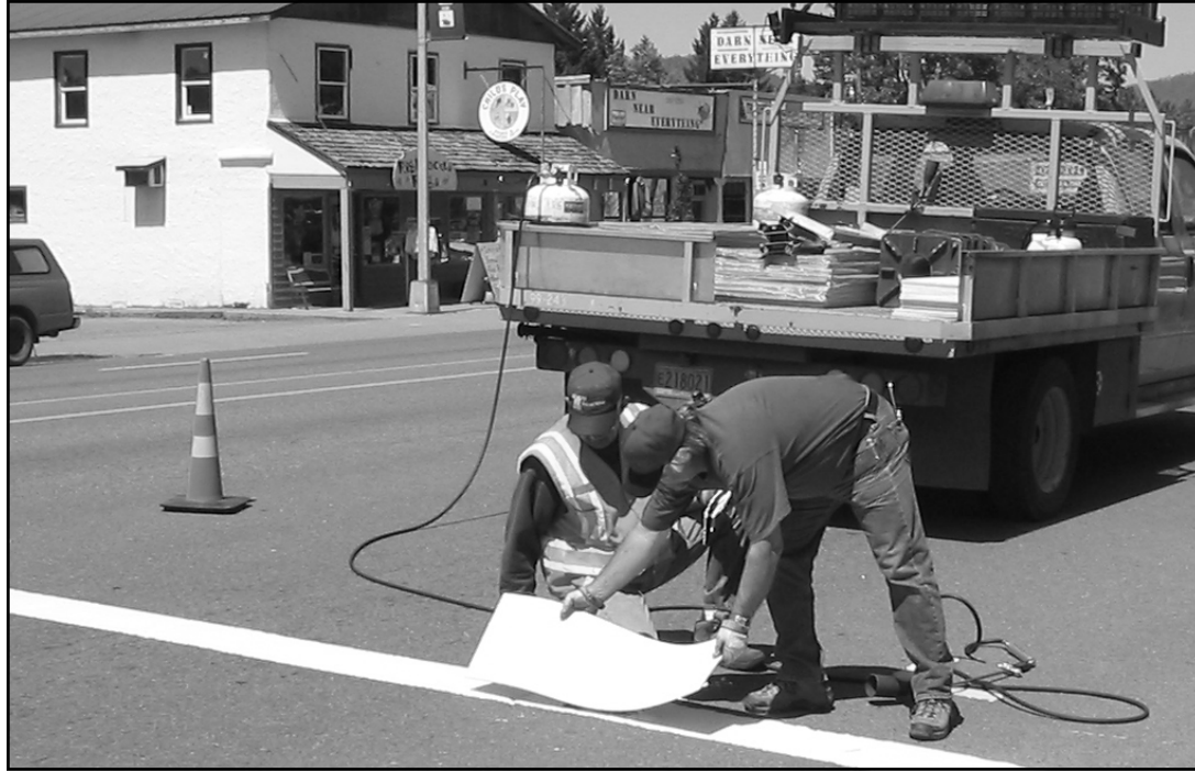
CJ CROSSWALKS RENEWED - Workers from the Oregon Dept. of Transportation perform routine maintenance to replace crosswalk reflection strips on Redwood Hwy. in Cave Junction on Wednesday, April 28. Using a large torch, workers heated the strips until they began to 'melt' and permanently stick to the pavement, making it easier for motorists and pedestrians to see the crossings. (Photo by Shane Welsh)
