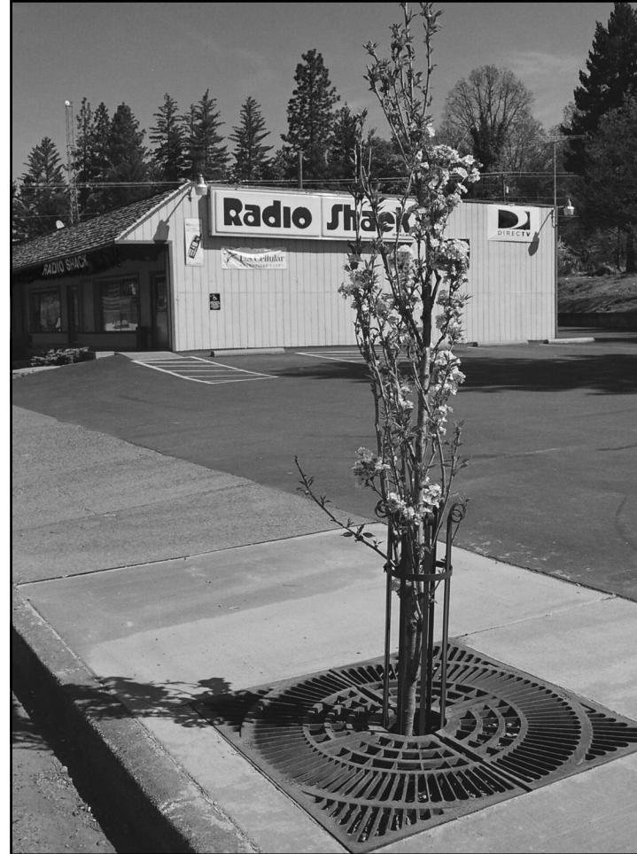
GRATE TREE - Some 20 flowering trees with decorative grates have been installed in Downtown Cave Junction as part of beautification that included removal of trees whose roots had pushed up sidewalks.
