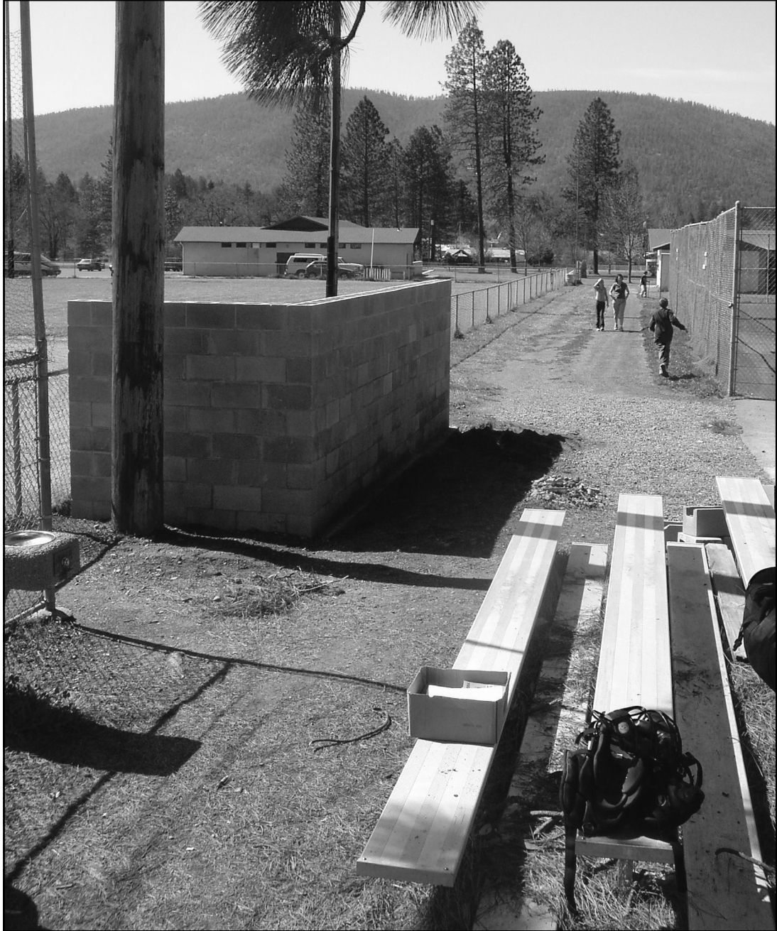
DANDY DUGOUT DELIGHT - Volunteers with Illinois Valley Little League continue to work to improve the ball field and related items at Jubilee Park. New dugouts are being built and are awaiting installation of roofs. Volunteers also are resurfacing the field in preparation for the start of the season on Saturday, April 10. The season opening ceremony will be on May 1.
