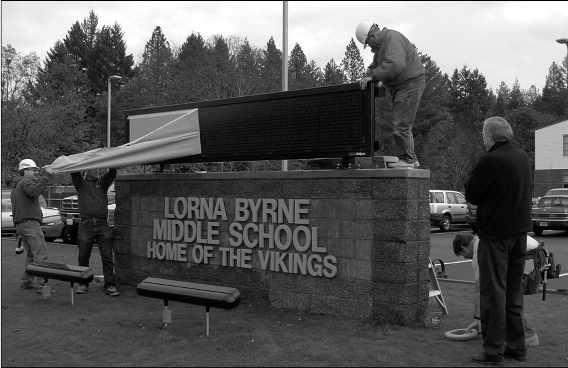
VIKING SIGN OF THE TIMES - Workers from Ashland-based Adroit Construction put the finishing touches on the entrance sign at the new and improved Lorna Byrne Middle School on Tuesday, Dec. 2. Adroit is the prime contractor for the $9.2 million overall project.
