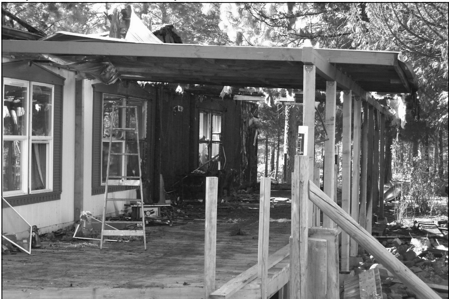
LONE MOUNTAIN FIRE -- Illinois Valley volunteer firefighters extinguished a blaze at the home of Sterling Goode at 552 Lone Mountain Road in O'Brien on Wednesday, Sept. 24 at 6:17 p.m. Smoke from the fire was seen by a Oregon Dept. of Forestry lookout on Grayback Mountain. The fire was deemed an electrical fire. The estimated loss caused by the fire was $150,000. (Photo by Steve Fairchild)
