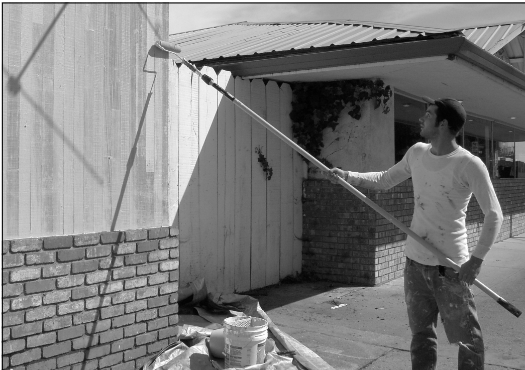
PAINTING THE TOWN -- David Holmes helps give a much needed face-lift with a fresh coat of paint to the outside of Bi-Rite Auto Parts located in the former Ivy Theatre in Downtown Cave Junction. (Photo by Britt Fairchild)
