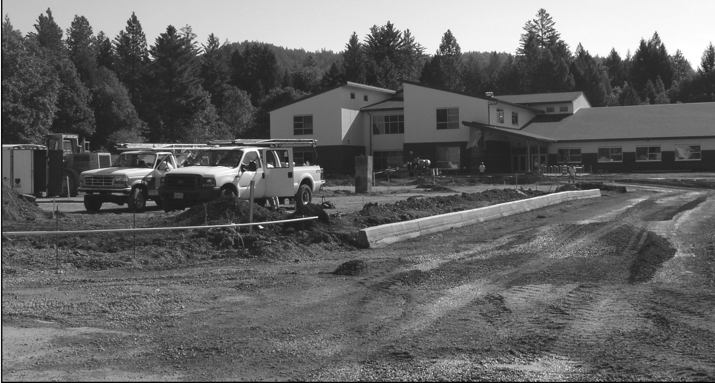
CONTINUING CONSTRUCTION - Lorna Byrne Middle School will soon be filled with students anticipating attending classes in their brand new school as they
